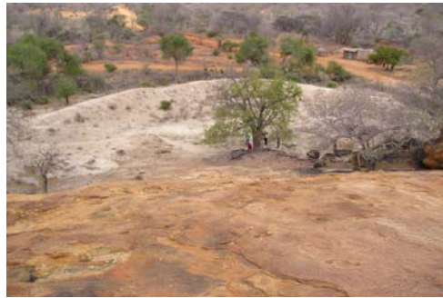
An earth dam built at a rock outcrop at Mutha in Kitui by ALDEV in 1958.
