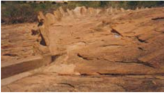
Garlands of stone gutters start their upward gradient (slope) of at least 3 cm per 100 cm from the end of a dam wall.
