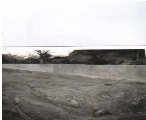
A filter/intake box with a non-return valve is placed in the deepest part of a rock pool in a rock catchment dam in Mutomo, Kitui.
