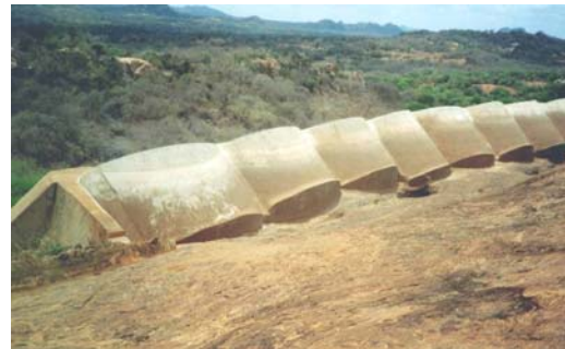
A complicated slanting multi-arch rock catchment dam at Mutomo.
