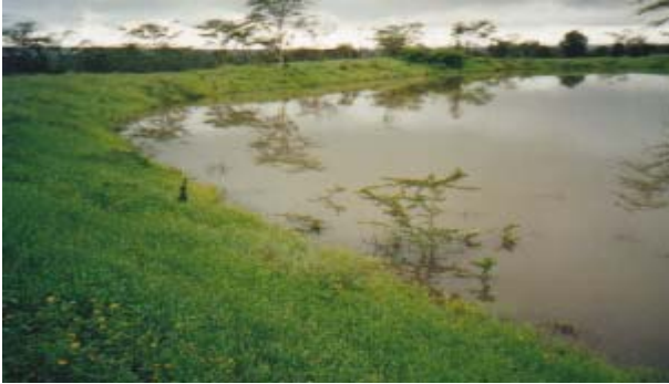
A curved hillside dam full of water from Lukenya Rock near Nairobi.
