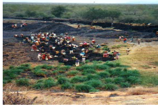
A self-help group desilting their curved hillside dam at a rock near Voi.
