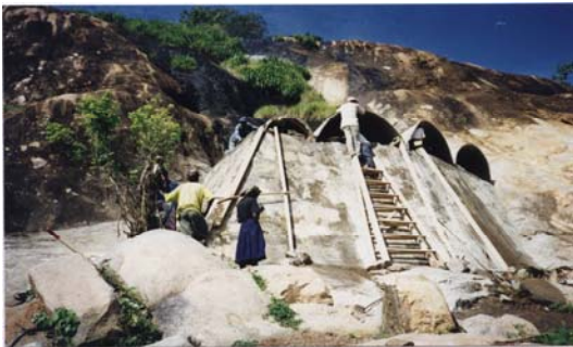
A rock catchment dam being roofed.
